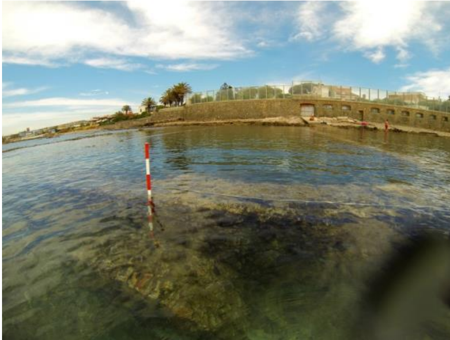
The fish tank of Punta della Vipera with the separation walls between the pools and the channel.
